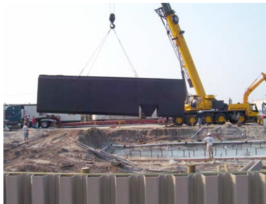
The Plant – delivered to the site
